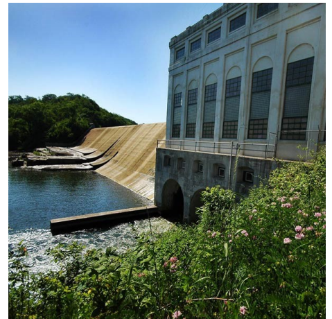
Zumbro Hydro Dam | Rochester Public Utilities
